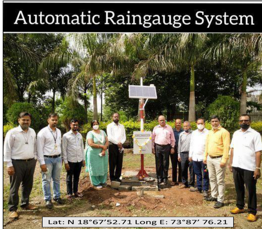
Automatic rain gauge system installation
