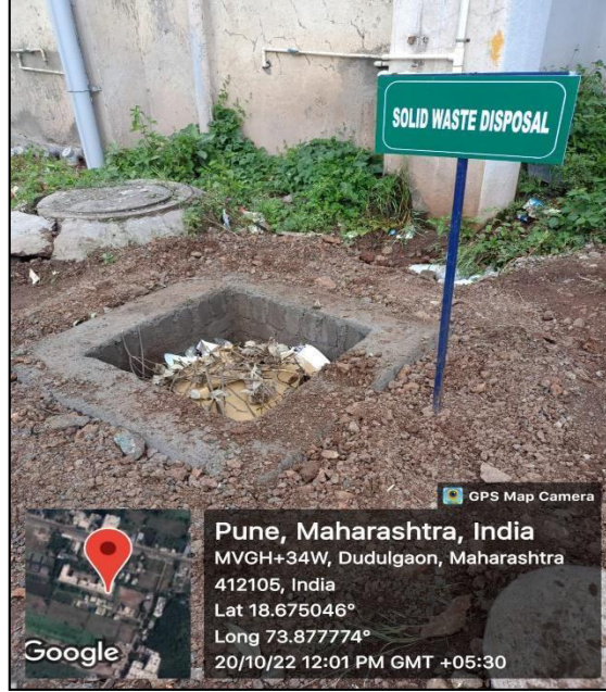
Solid waste disposal by compost pit
