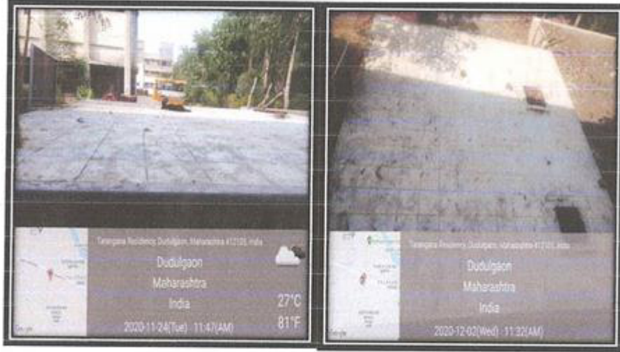
Water Storage Tank
